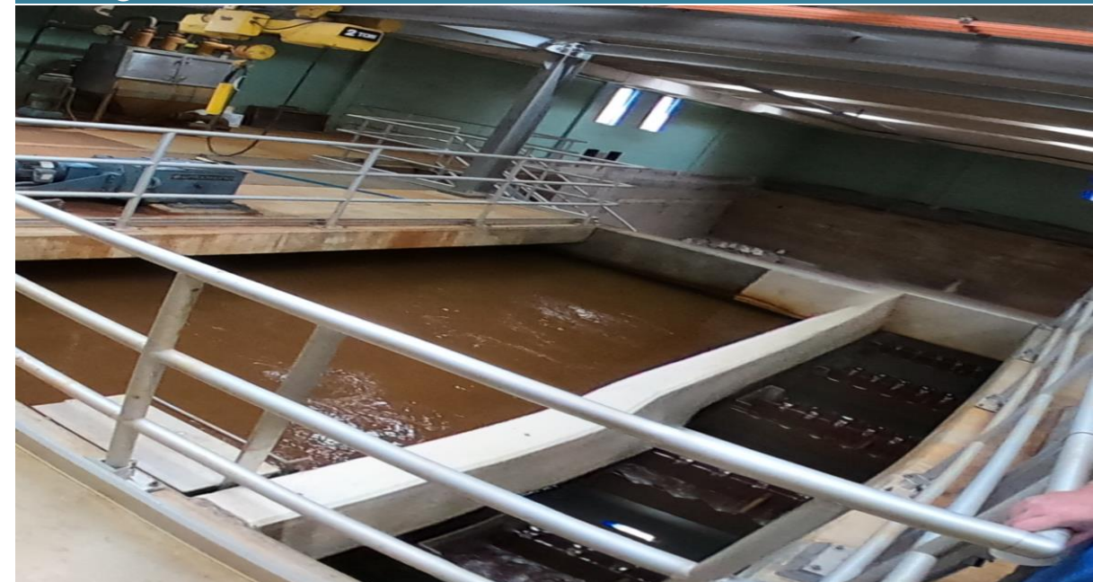
CWRWS Water Treatment Plant, Casper, WY
